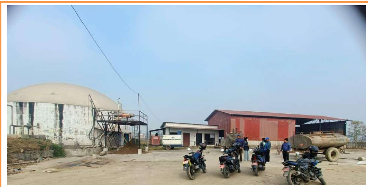
Photo No. 1. Biogas Plant Area
